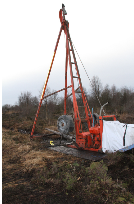
Plate 3-1: Shell and Augur borehole excavation on site
