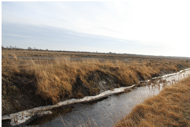
Plate 3-3: The main drain at the northern edge of the bog which ultimately receives surface waters from drains across the site, and links to the River Barrow. This was characterised by no obvious flow (ice covered), clear water (despite heavy recent rain), patches of bulrush Typha latifolia (vegetation cover) and a very flat topography. No evidence of excessive silt runoff was recorded as a result of the site investigation works or other nearby activities.
