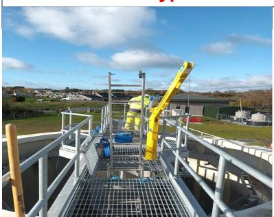
Typically access into concrete tanks were via access installed on bridge/ walkway floors or via gates and ladder supports incorporated bridge/ Walkway Handrailing
