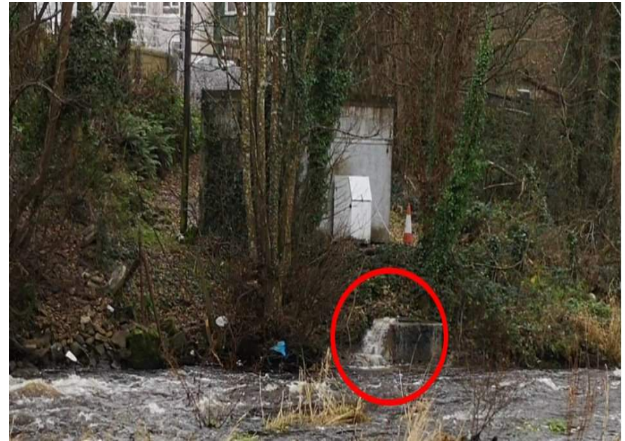
Overflow at Pumping Station adjacent to the N67 Lahinch Road into Inagh River during heavy rainfall events. Pumps and pipelines have insufficient capacity to deal with these events
