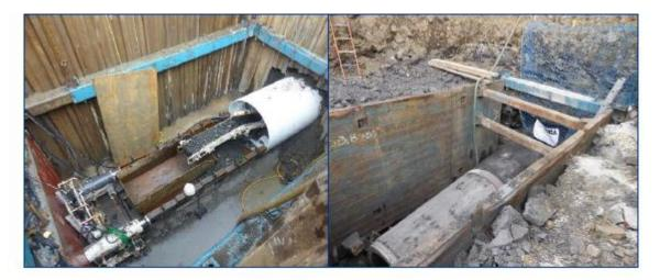
Figure 16: Tunnel Jacking Launch Shaft
