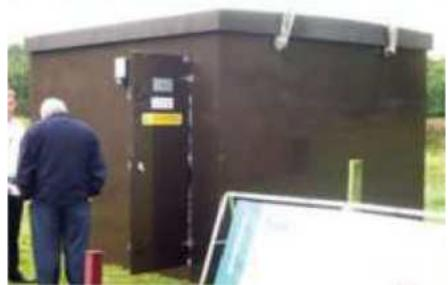
Figure 5 Typical orthophosphate dosing unit
