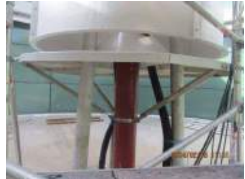
Figure 3.16: McKinney Baffle
