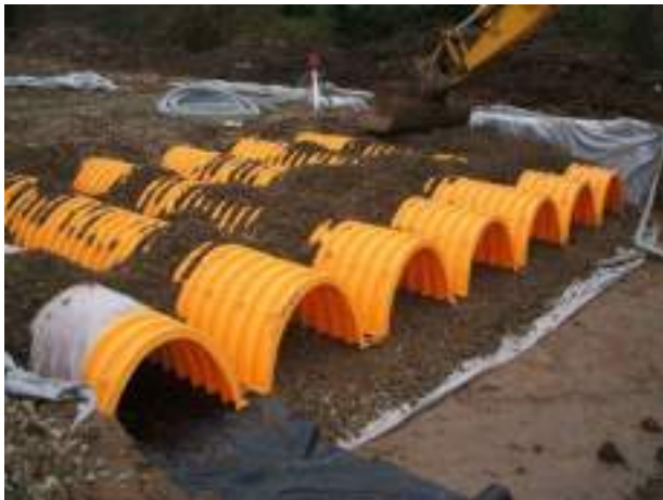
Figure 3.24: StormTech Storm Storage Tank
