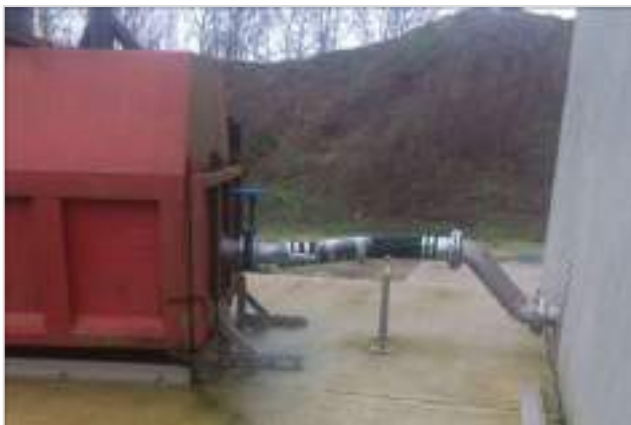
Figure 3.19: Enniscorthy WwTP Dewatered Sludge Storage
