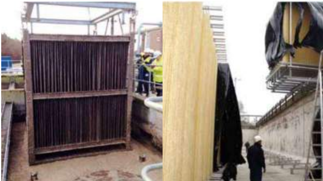
Figure 3.11: Example of IFAS frames and textile curtains (courtesy of Eliquo Hydrok, Appendix 2A)
