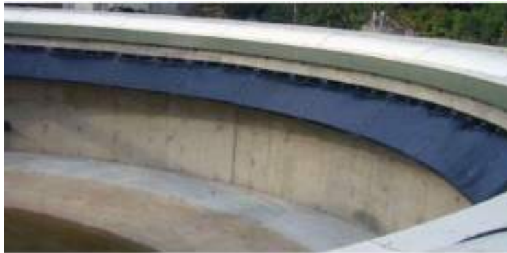
Figure 3.15: Stamford Baffle
