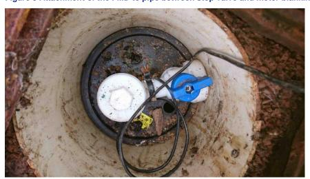
Figure 3 Attachment of the FMD to pipe between stop valve and meter blanking plate
