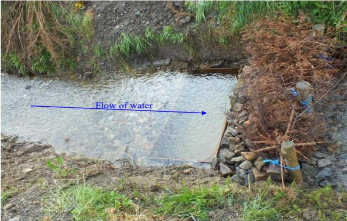
Figure 7 Silt trap installed in stream at Kilberrihert
